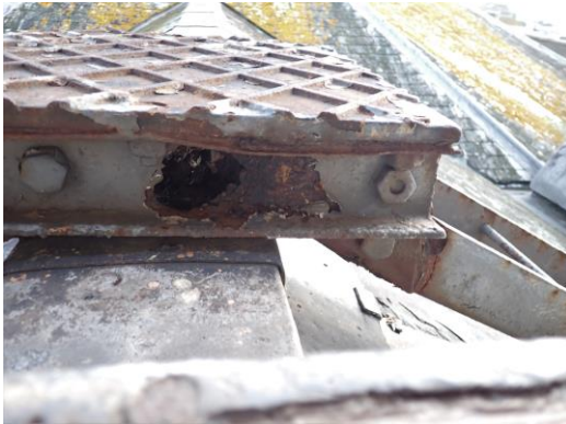
Main roof access platform
