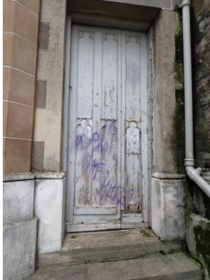
East door of South Porch
