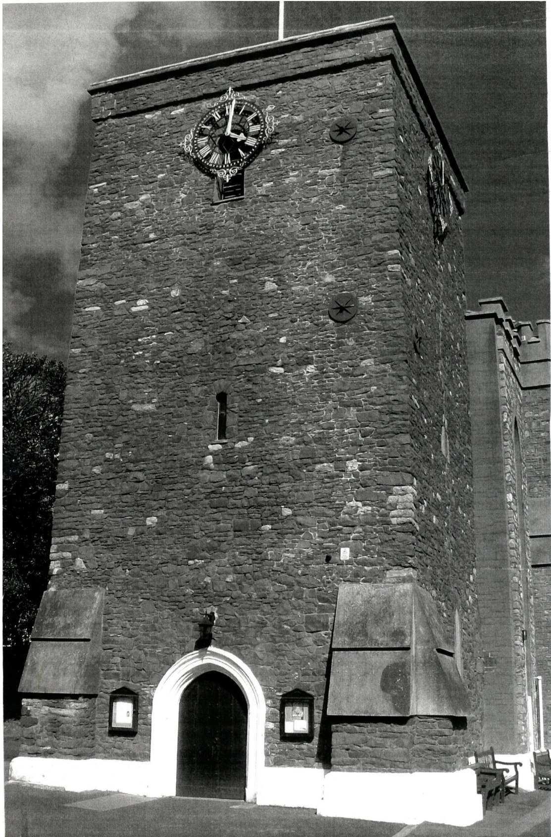
Fig 2. St James, West Teignmouth: west tower from west
