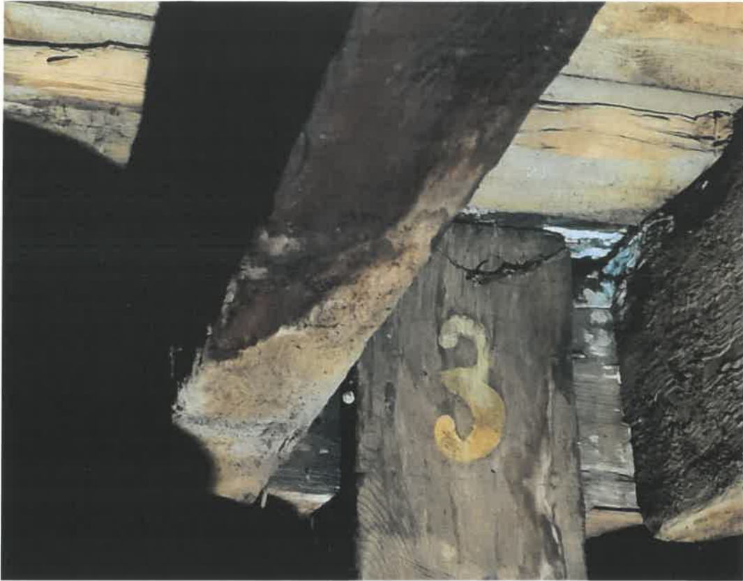
69 Rot to Roofing Boards
