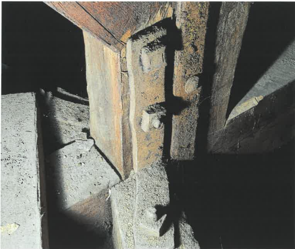
68 Ironwork to Truss
