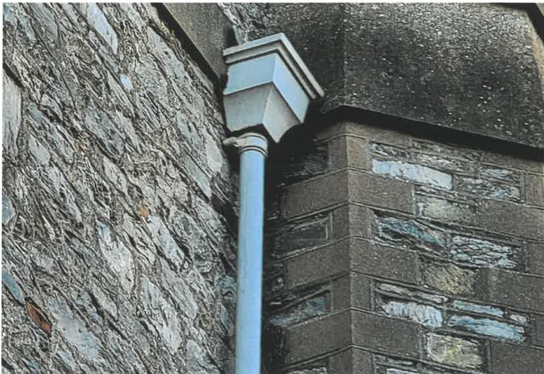
14 Hopper in Reasonable Condition
