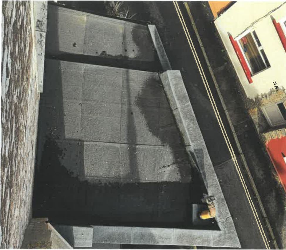
11 Vicar's Vestry and Toilet Roof
