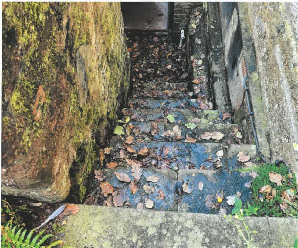
64 Steps to Boiler Room
