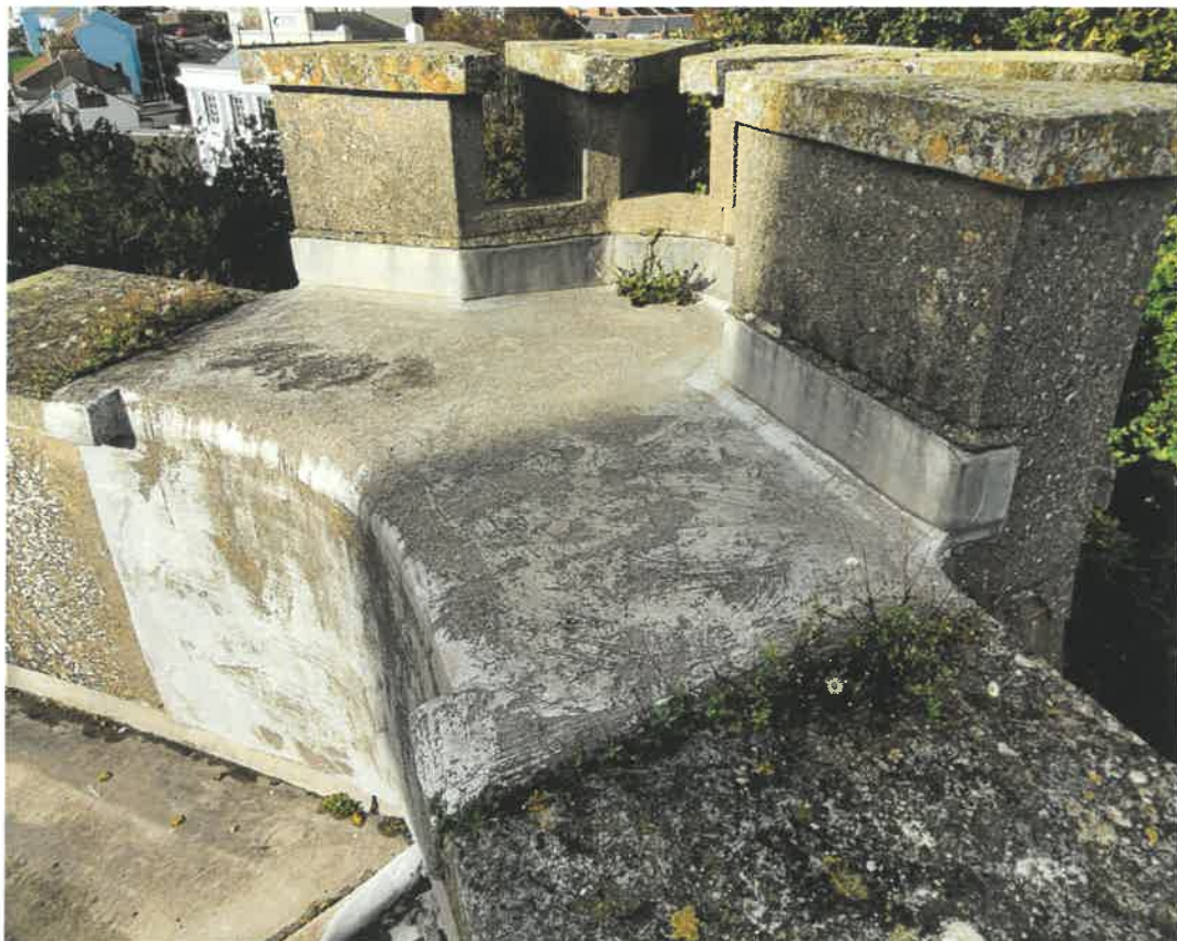
18 Battlement to Main Roof
