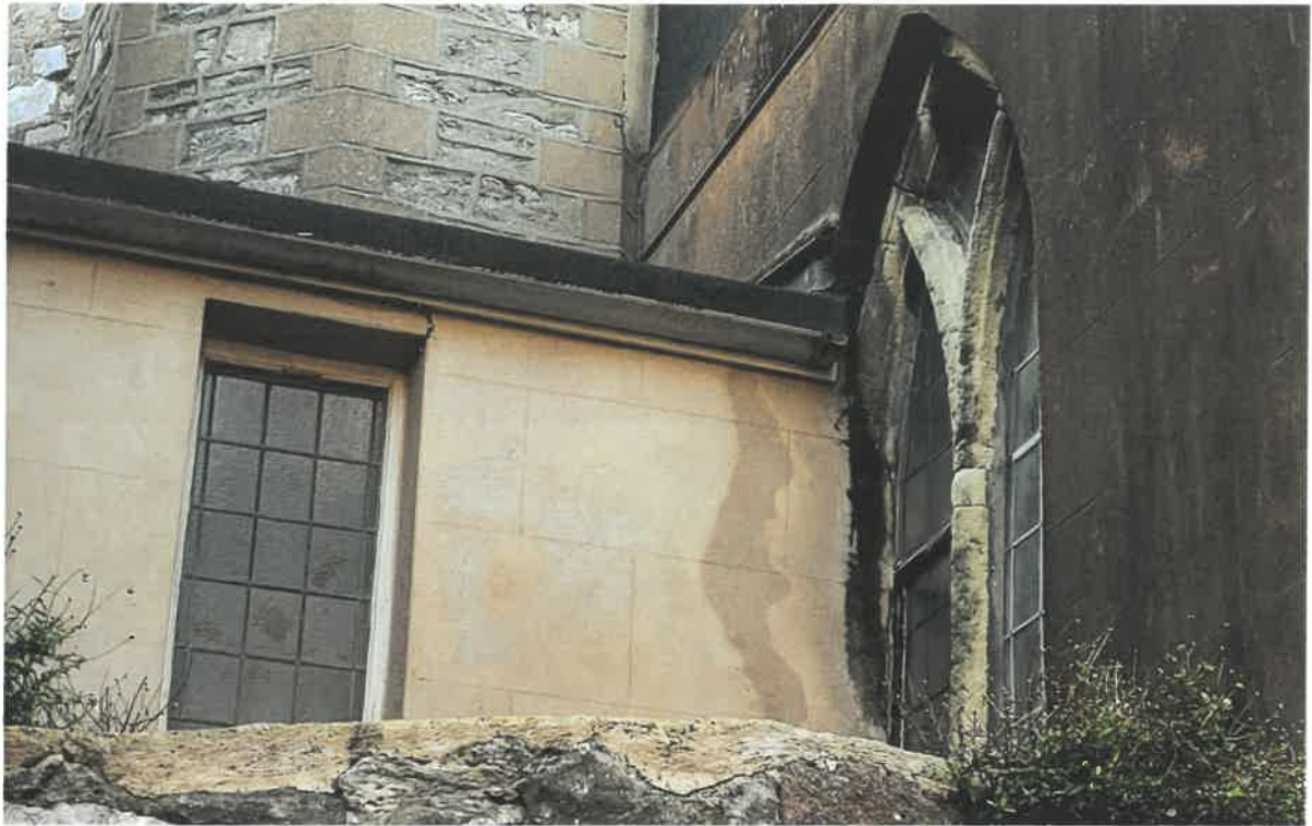
33 Windows W2 and W3
