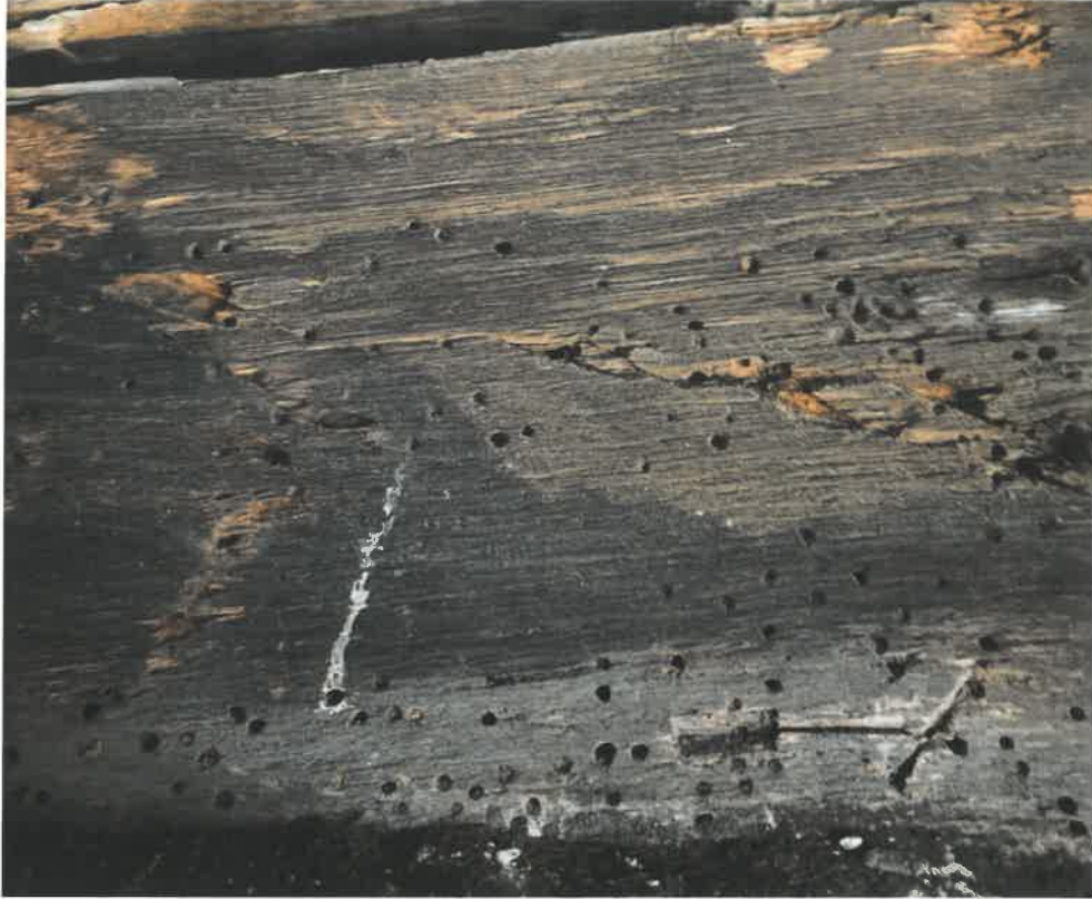
63 Tower Roof Beam
