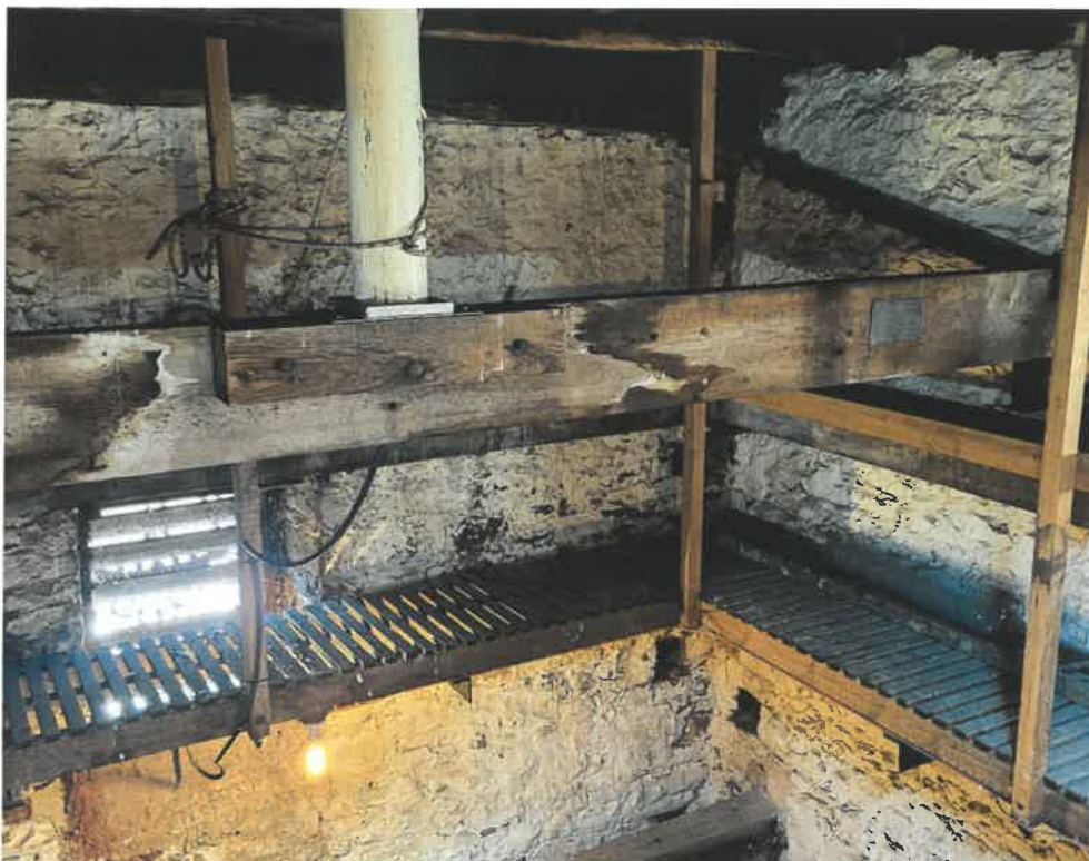
62 Bell Chamber Gantry
