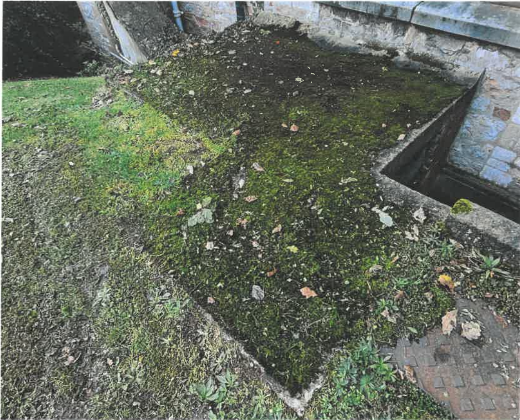
13 Boiler Room Roof
