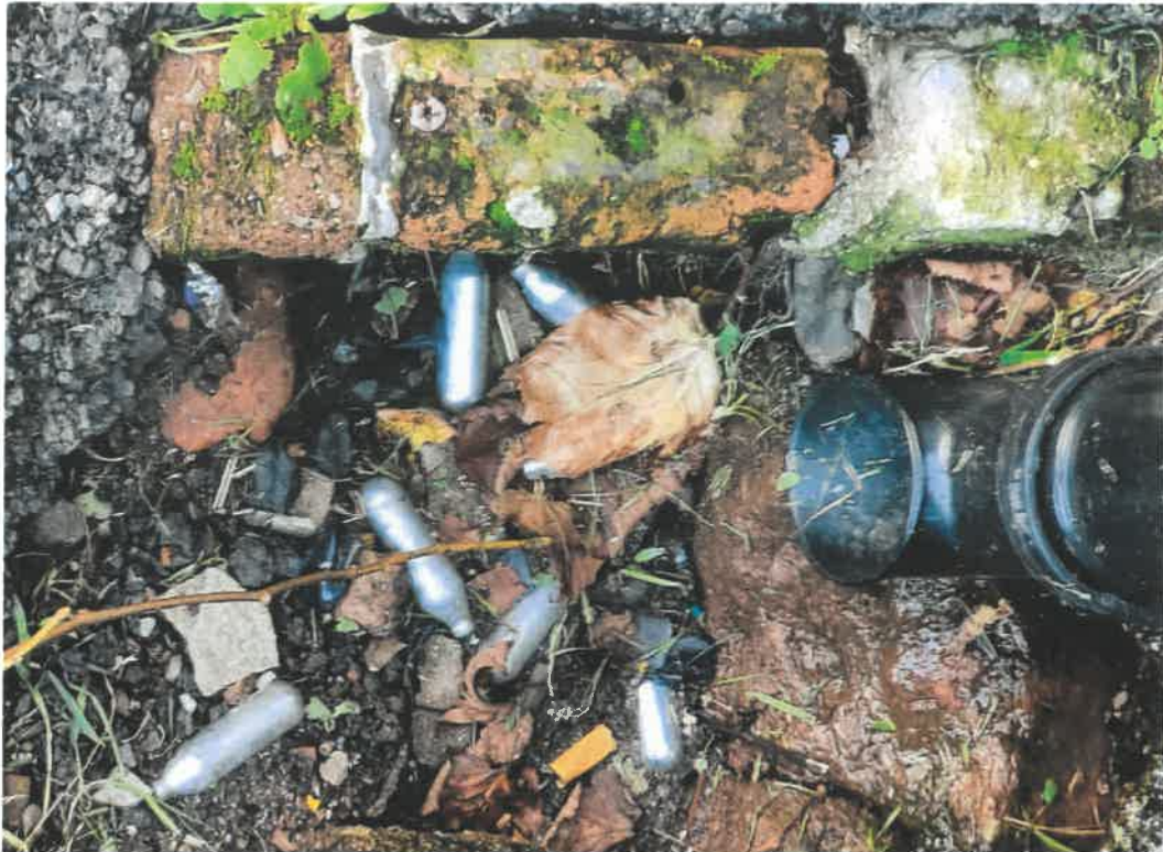
17 South Porch Gully
