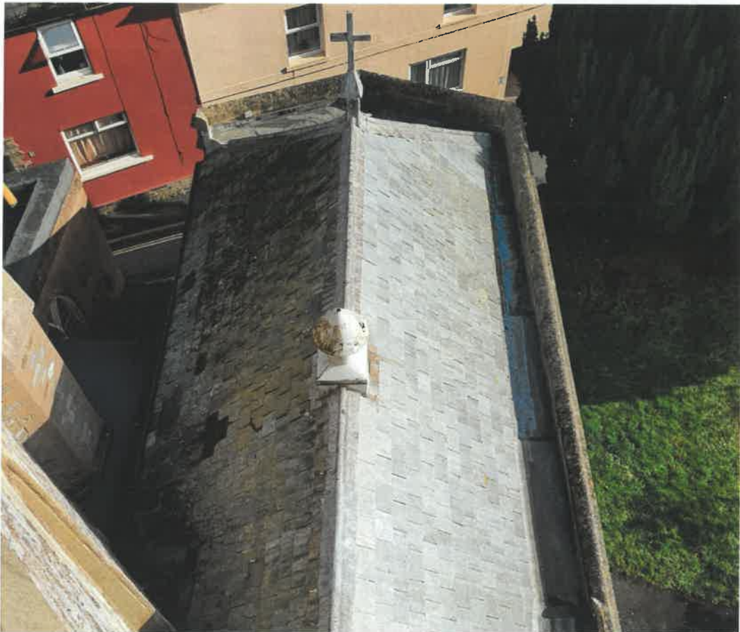
10 Whitford Room Roof
