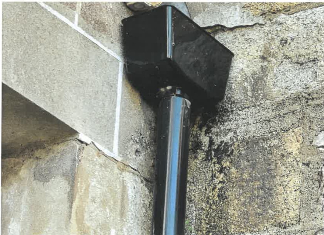
16 South Porch Hopper and Rainwater Pipe
