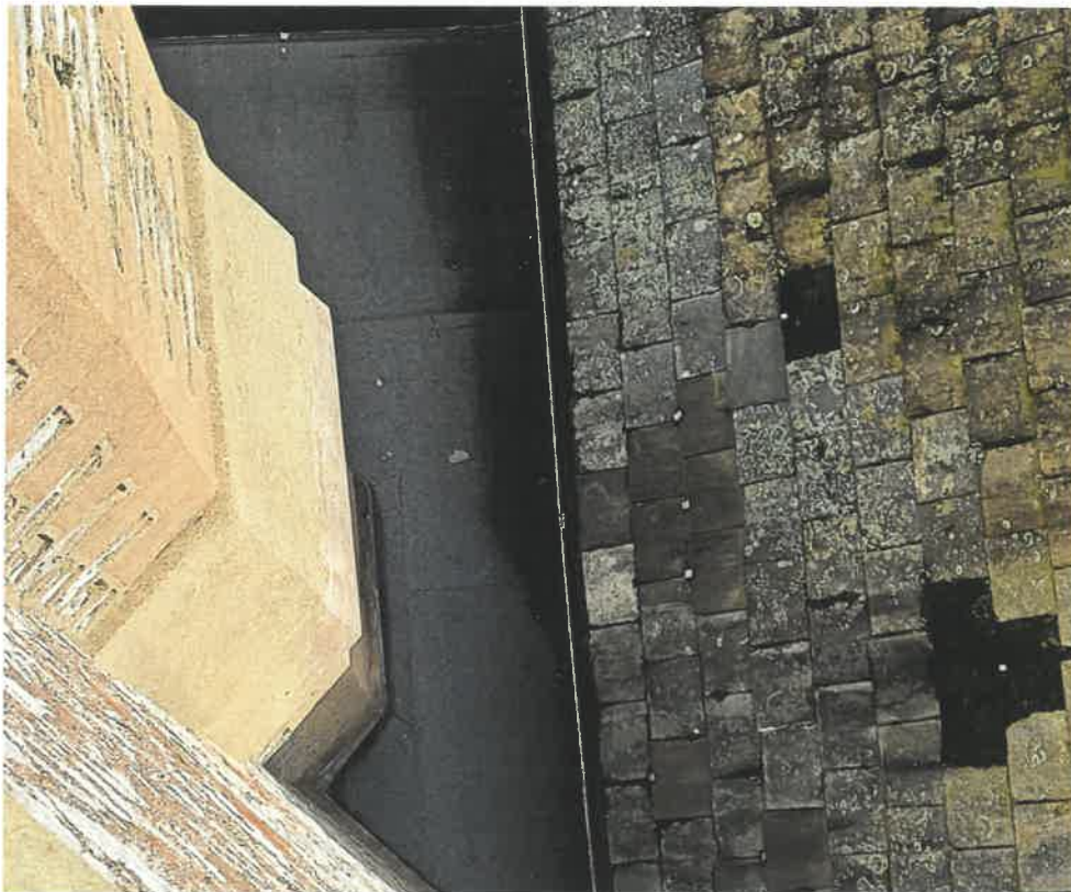
12 Link Corridor Roof
