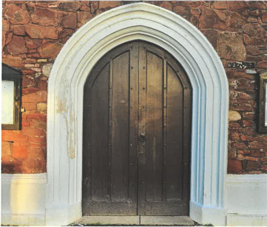
27 Door D1 – Tower
